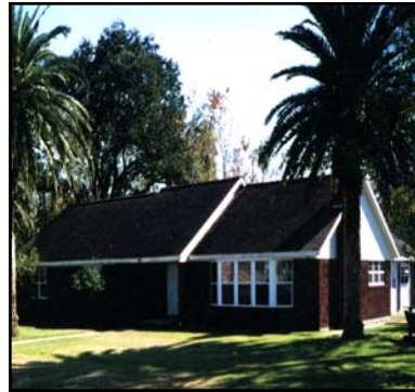
New Facility in Texas City
